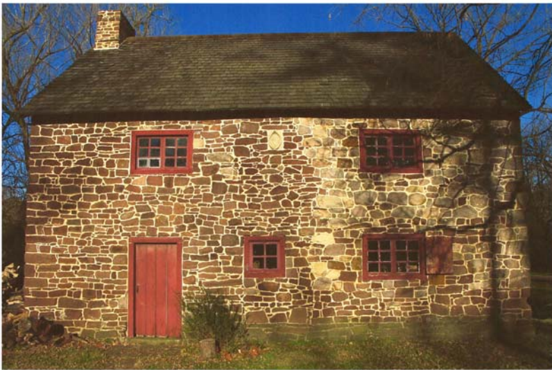
Mouns Jones House (1716) - West Eaves Wall (to be restored) 2013
